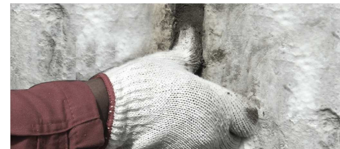
Injection>> Removing packers>> Closing packer holes
