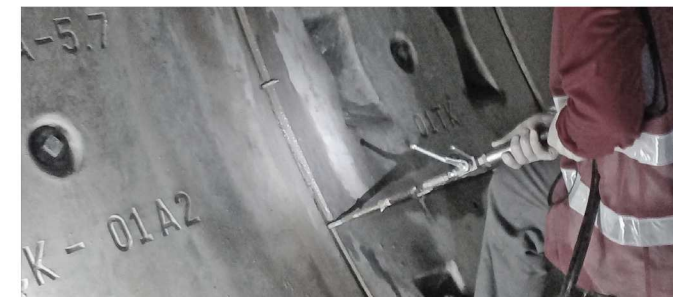
Injection>> Removing packers>> Closing packer holes
