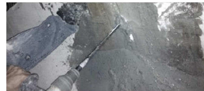
Drilling hole>> Removing dust and dirt
