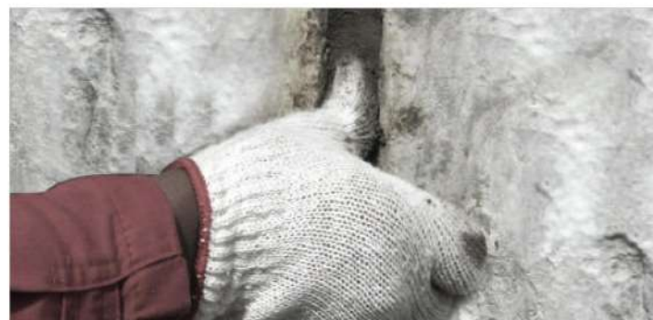
Injection>> Removing packers>> Closing packer holes
