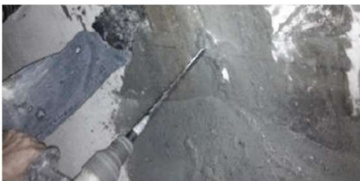
Drilling hole>> Removing dust and dirt
