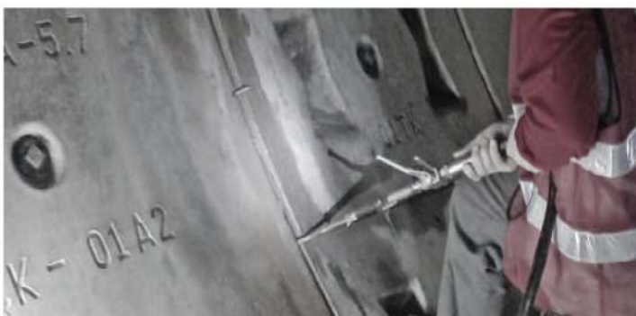
Injection>> Removing packers>> Closing packer holes
