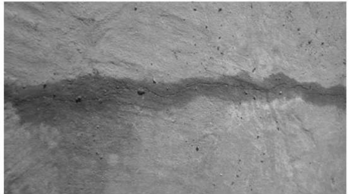
Water tank / Diaphragm wall
