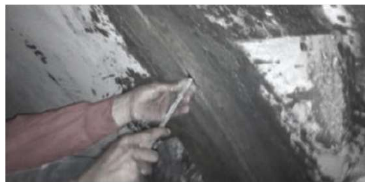
Tightening and fixing packers
