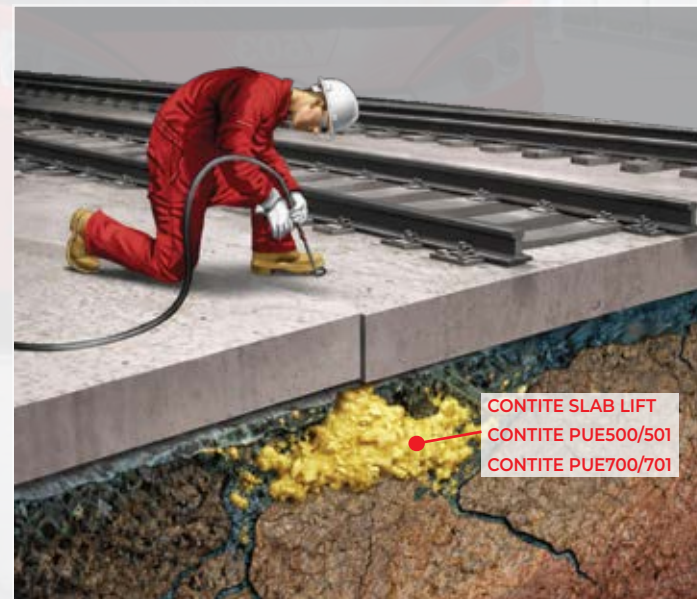
Rail Crossing Realignment with Rigid Foam
