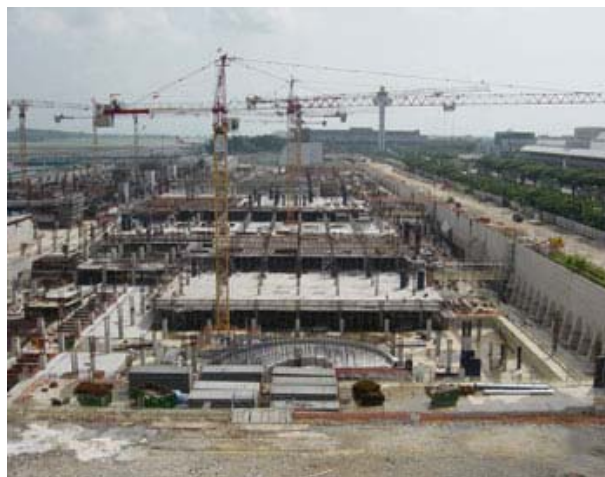
Basement Waterproofing Wastewater & Potable Water Tank Waterproofing
