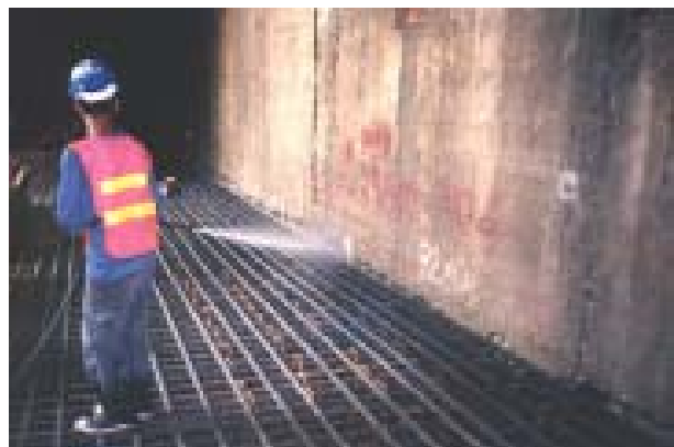
Surface preparation/cleaning by water blasting
