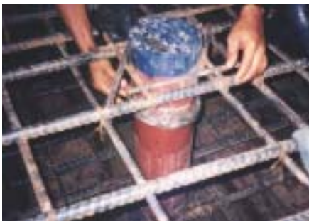
Installing Contite Waterstop Around Pipes
