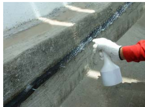
Contite Waterstop Delay Coating application by spray
