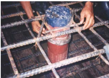
Installing Contite Waterstop Around Pipes
