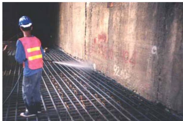
Surface preparation/cleaning by water blasting
