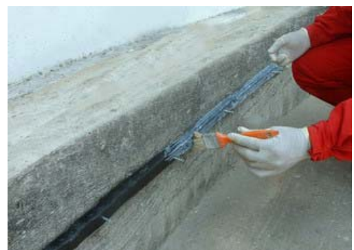
Contite Waterstop Delay Coating application by brush
