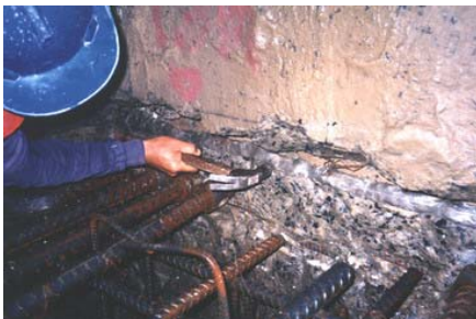
Nailing in place Contite Waterstop to rough surface
