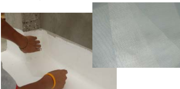
Elastoclad applied over existing roof membrane system.
