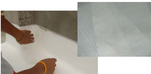
Elastoclad applied over existing roof membrane system.
