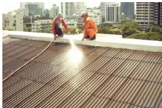
Application of Elastoclad by Spray
