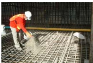
Dry shake to lean concrete
